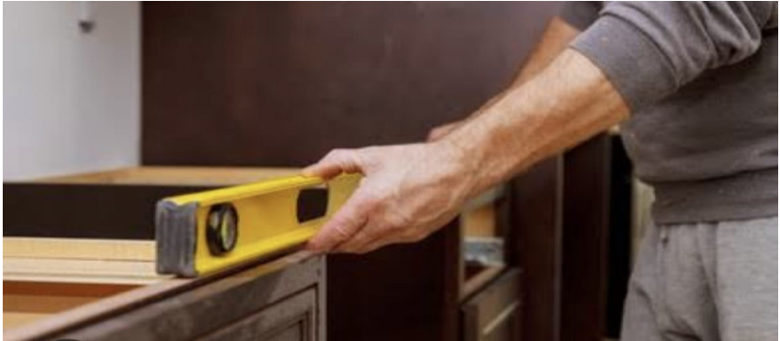
Fig:- (d) verifying counter alignment for precise levelling.
