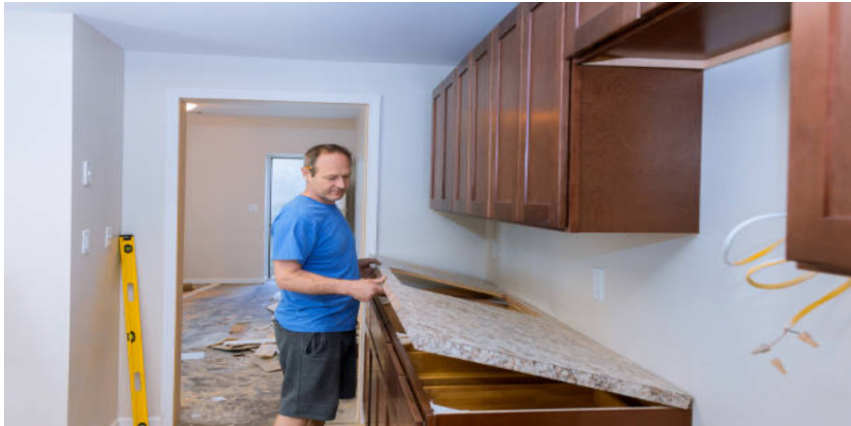
Fig:- (b) Ensuring the slab is perfectly sized for precision and fit.
