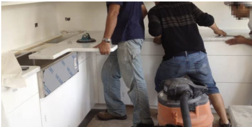
Fig:- © Ensuring the slab is perfectly sized for precision and fit.
