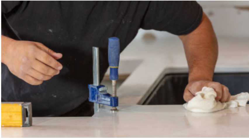
Fig:- (g) Clamp quartz slab securely for stability.
