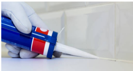
Fig:- (j) Apply silicone for sink and corner sealing, preventing water penetration.
